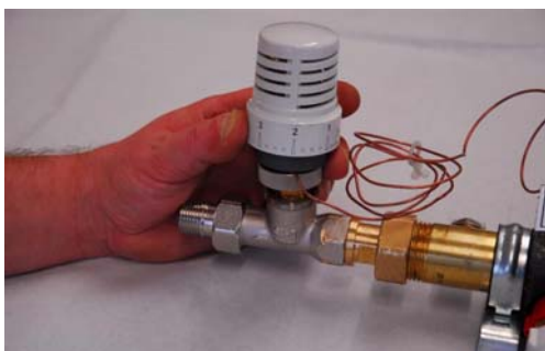
Step 2: Loosen the knurled screw and remove thermostat
